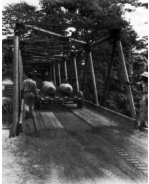
STEEL BRIDGE OVER THE LALOKI near Port Moresby, built in three weeks by an engineer company, November 1942.
